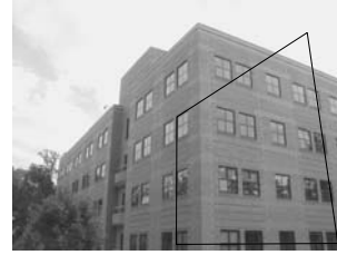
Figure 3. An example where the intersection of extended lines is outside the rectangular structure.
